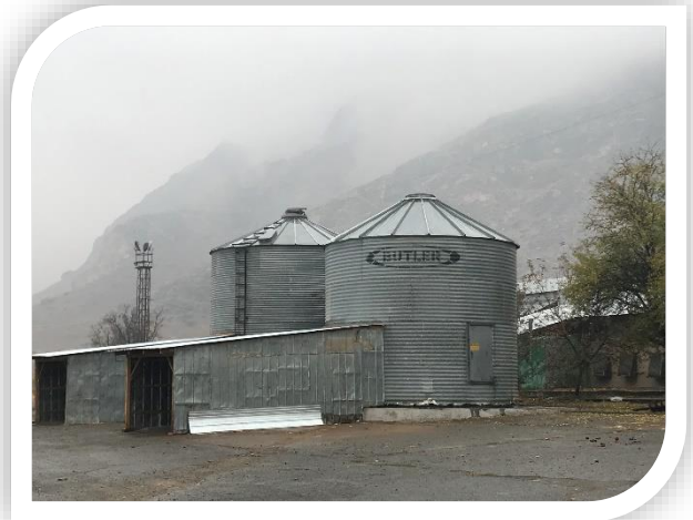
Grain bins built in Kyrgyzstan that had been sent from Palco, KS
