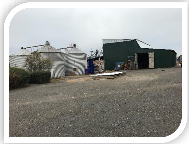
Feed mill and grain storage facility being supported in Kyrgyzstan
