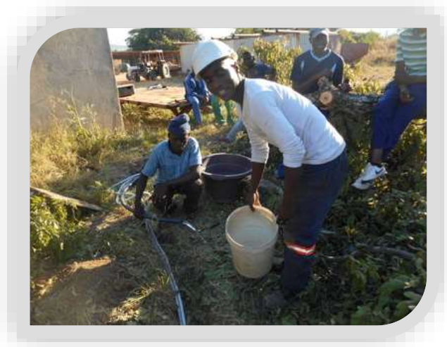
Water from a solar pump we funded in Zimbabwe.
