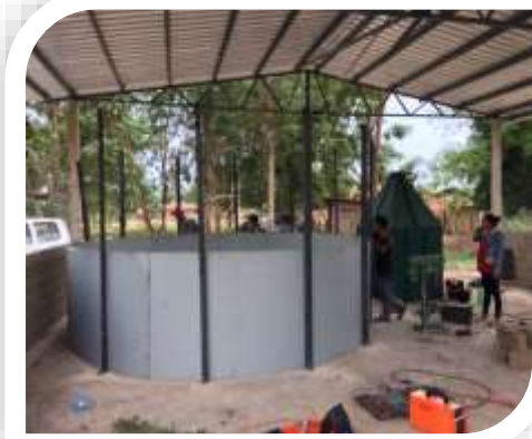
Harvest Center under construction in Laos
