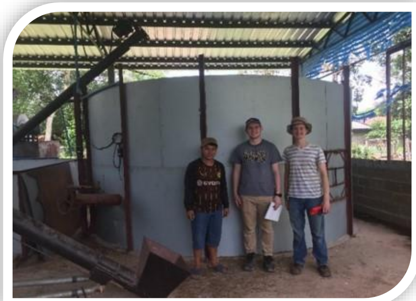
A harvest center being constructed in Laos
